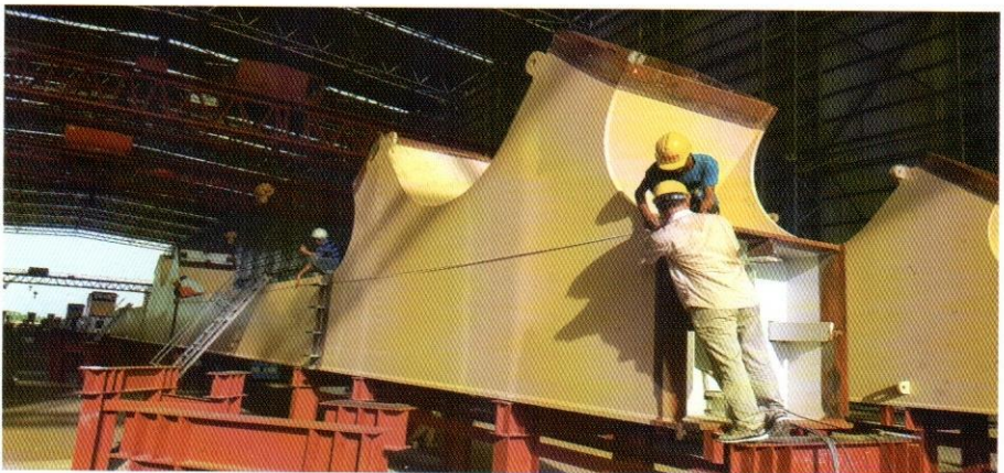
Dimension Inspection after fit-up
