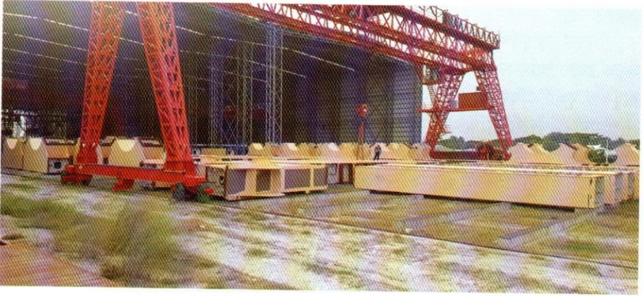
Storage condition of Node/Chord members – 1
