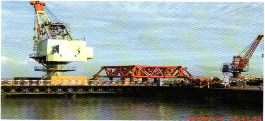
Fabrication of Cofferdam for River Span
